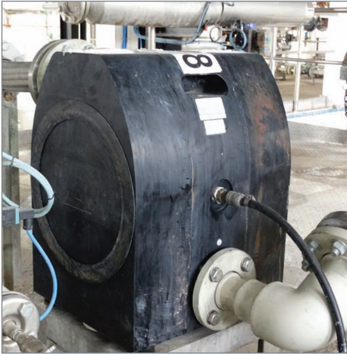
An E-50 model from the Almatec® E-Series AODD Pump family is used to safely and reliably transfer titanium dioxide (TiO 2 ), a powder used to make pigments for cosmetic and health-care products.
