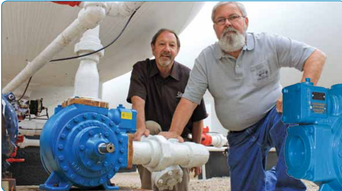
Steve Ward (left) of Gardner Marsh and Rickey Watkins of Apex Propane Services next to the new Blackmer LGL3021 sliding vane pump at the Apex bulk plant.
