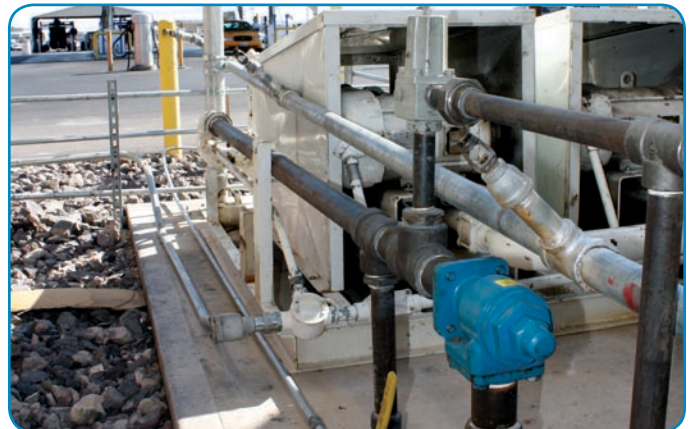
Blackmer BV2 Bypass Valves were also added to the fueling system.
