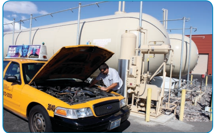
Kevin Ash, Supervisor – Propane Specialist for YCS, uses the vapor-recovery system designed by Blackmer distributor Meeder-Ransom to draw down the vapor level in the taxi prior to service. The vapor-recovery system features a LB161 Series compressor.
