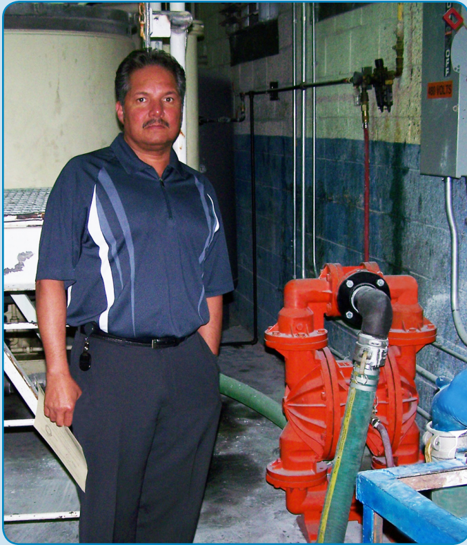
Santos Flores, Director of Corporate Maintenance for Diversified Chemical Technologies, Inc., next to one of the many Wilden AODD pumps that have helped him stimulate the bottom line by reducing downtime by 50%.
