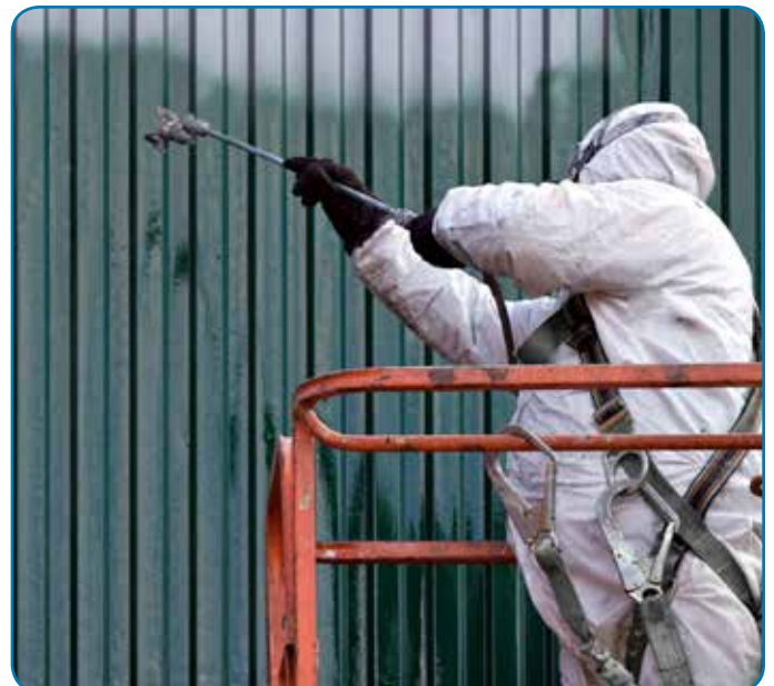
In order to improve energy efficiency in paint & coatings facilities, operators are utilizing energy optimization programs, such as Blackmer's Smart Energy Flow Solutions.
