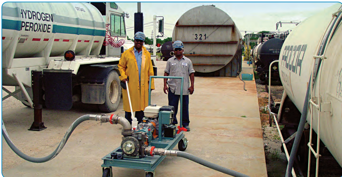
Operators at this chemical distribution/storage terminal facility transload hydrogen peroxide from a railcar to a transport via a Blackmer sliding vane pump.
