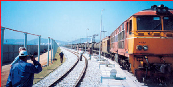
Rail tanker bulk unloading facility
