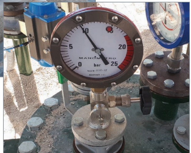
The decision to use an Ebsray® RC40 Series pump, in white above, in EWAPPOINT's new Autogas installation in Santa Maria Capua Vetere hinged on its ability to reliably create 10 bar (145 psi), right, of differential pressure during its operation. That much differential pressure is needed to ensure a smooth-running fueling process, especially in the hot summer months that are common in southern Italy.
