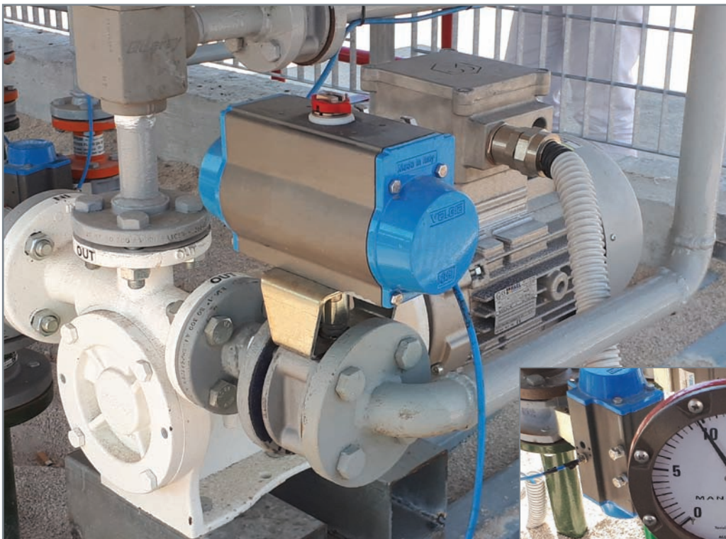
The decision to use an Ebsray® RC40 Series pump, in white above, in EWAPPOINT's new Autogas installation in Santa Maria Capua Vetere hinged on its ability to reliably create 10 bar (145 psi), right, of differential pressure during its operation. That much differential pressure is needed to ensure a smooth-running fueling process, especially in the hot summer months that are common in southern Italy.
