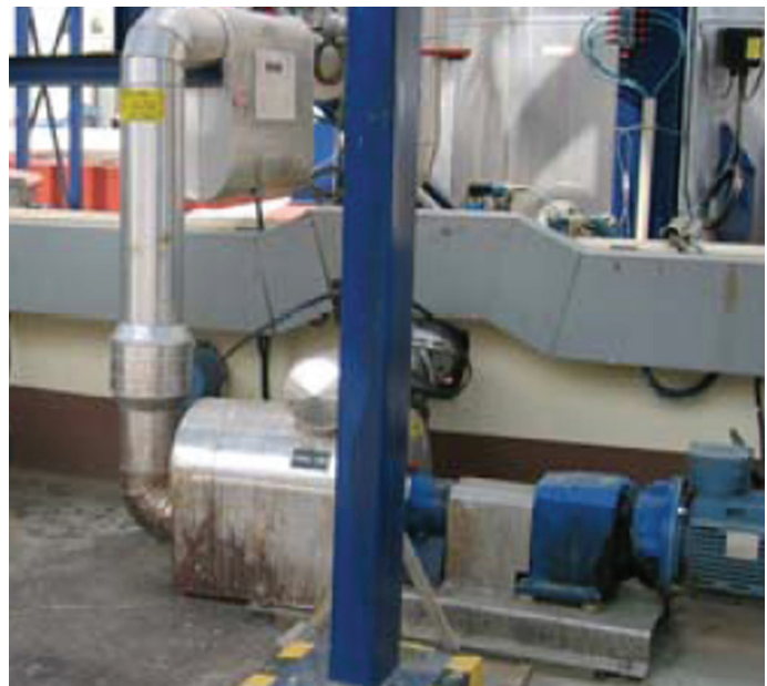
This eccentric disc pump has successfully handled polyurethane paints made from MDI at an automotive paint plant since 2001.
