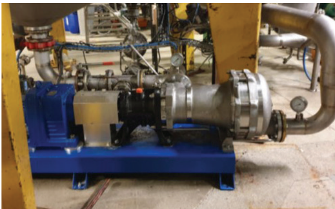
Eccentric disc pumps are successfully handling flocculent at a polymers plant.
