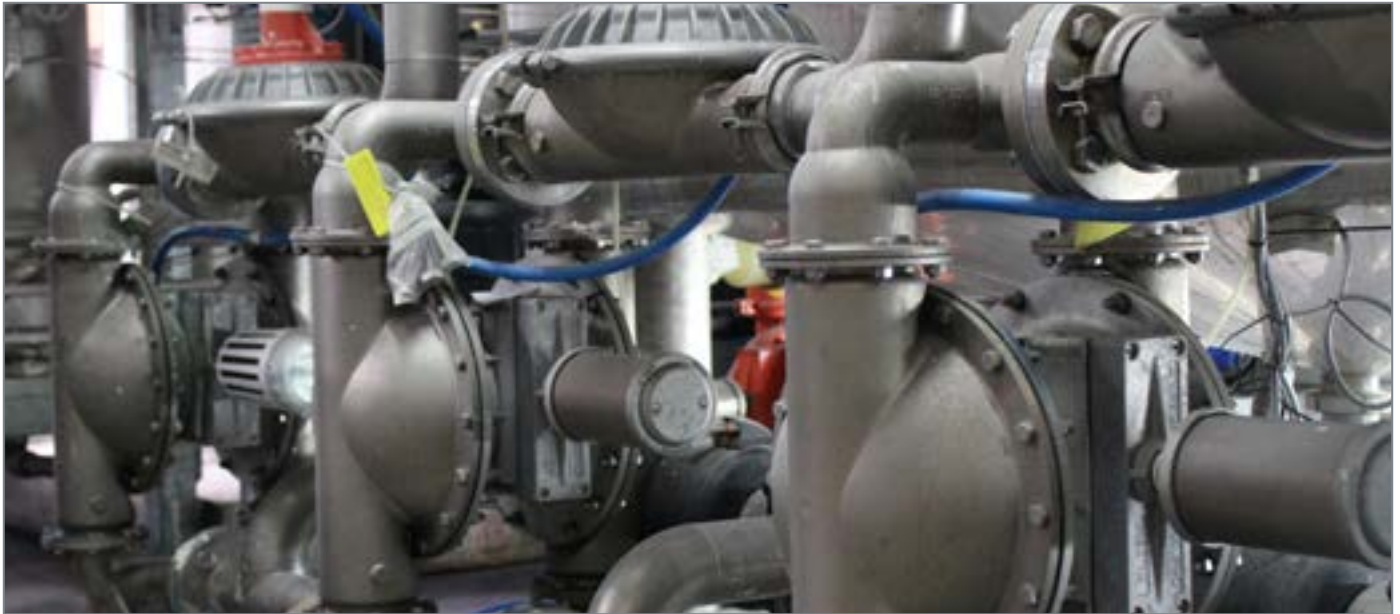
Wilden® Clamped and Bolted AODD pumps are the perfect solution for Havo thanks to their ability to handle high-viscosity liquids. Additionally, Wilden pumps feature a redesigned liquid path that reduces internal friction for maximized flow rates and pumping efficiency.
