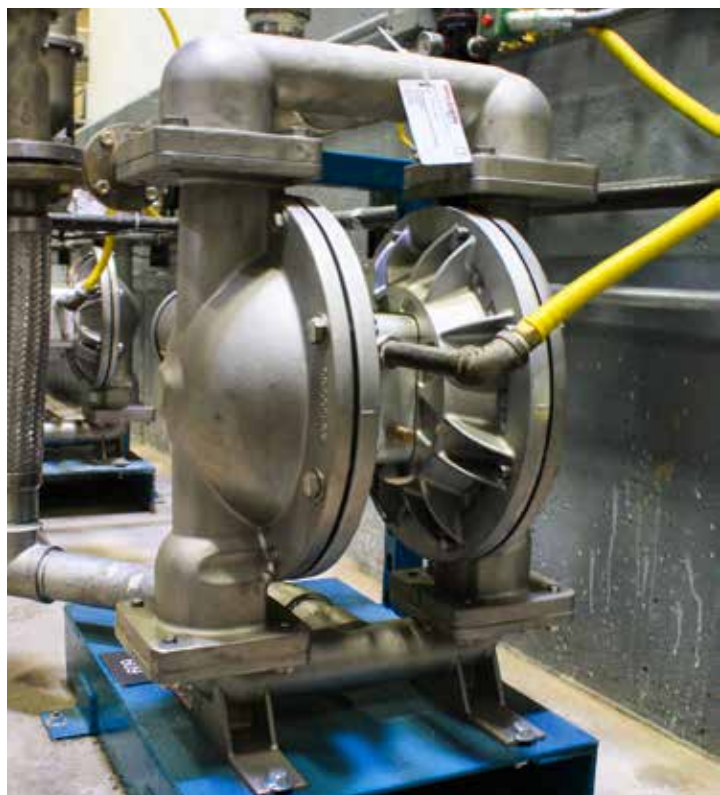
Image 1. While plastic pumps are typically a go-to pumping technology in chemical processing, there can be instances where metal pumps are a better choice for the operator. (Images courtesy of Wilden)
